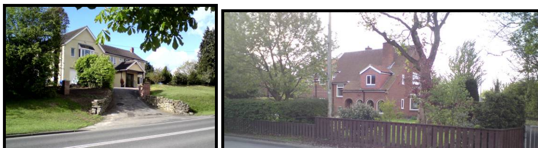
Images: 20 Leven Road and 6 Leven Road
