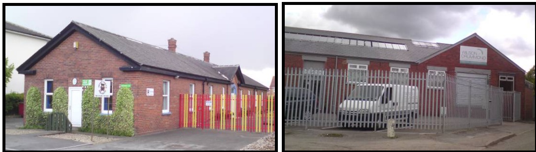
Images: Barrack Block and Stores and Workshop
